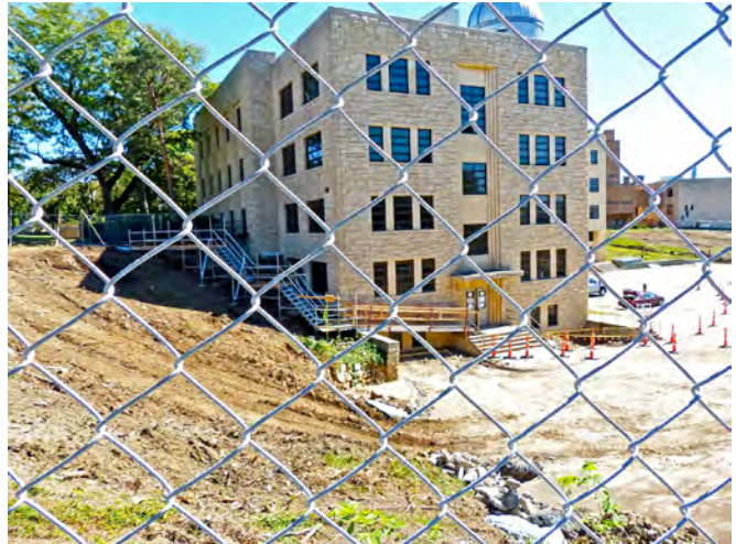
This view on October 2, looks at Lindley Hall through the newly erected fence, which now surrounds both parking lots.
