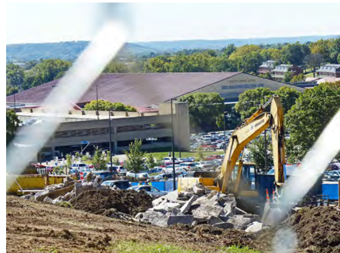
That pile of cement is all that remained in early October of the sidewalk and steps that once led from the Art and Design Building.
